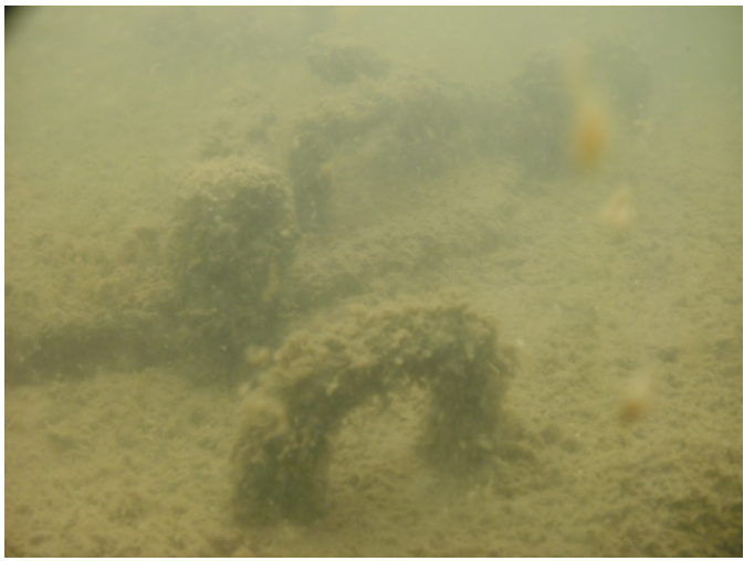
Photograph 7. Manhole 35 lifting eye.
